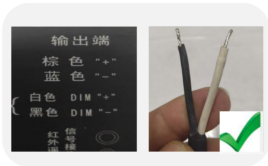
Correct wiring, normal lighting
