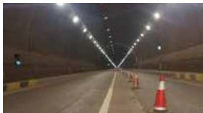
#2322 IESNA Type II Short Vertical (iso-brightness) lighting distribution
